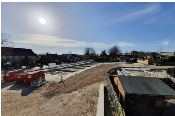
Start bouw in Hardenberg
